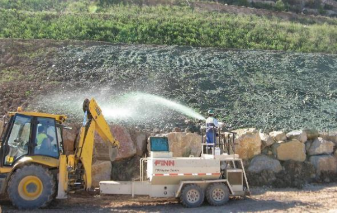
Hydroseeding in slopes
